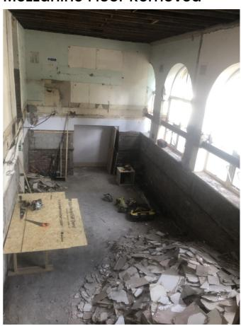
"Looking down into the space that will be the Market Hall. The dividing wall on the left is still to come down. The back wall shows shadows of the kitchen cupboards in the River Room kitchen. Rooms 1-4 on the ground floor have gone. The girder that used to support the mezzanine floor can be seen across the windows.
